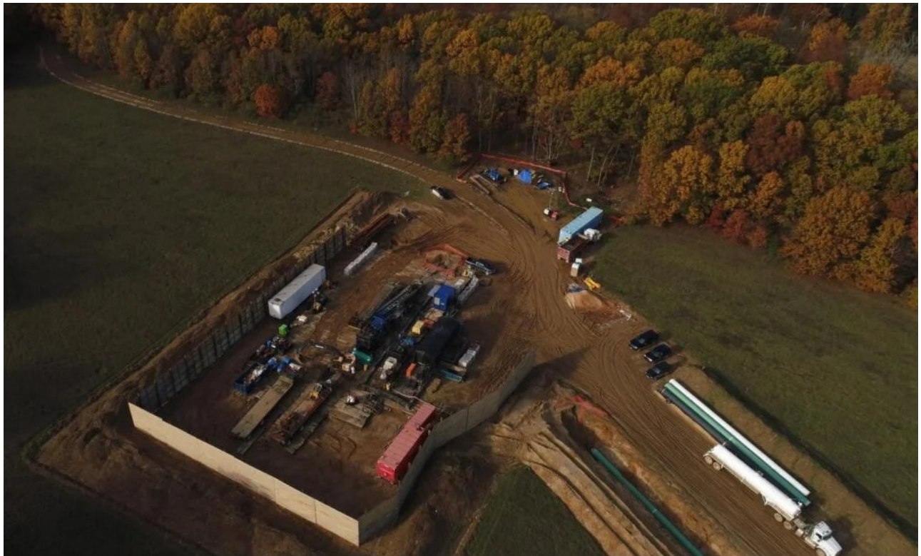
Images show: The drone footage shows the “rig side” of an active HDD site. Note the tall metal walls that surround the work site; the large security presence (in the black pickups), the matting that is underneath much of the equipment, and the blue pipeline that is sitting in the trench and the un-assembled pieces of blue pipe sitting on the surface (on the right side).
