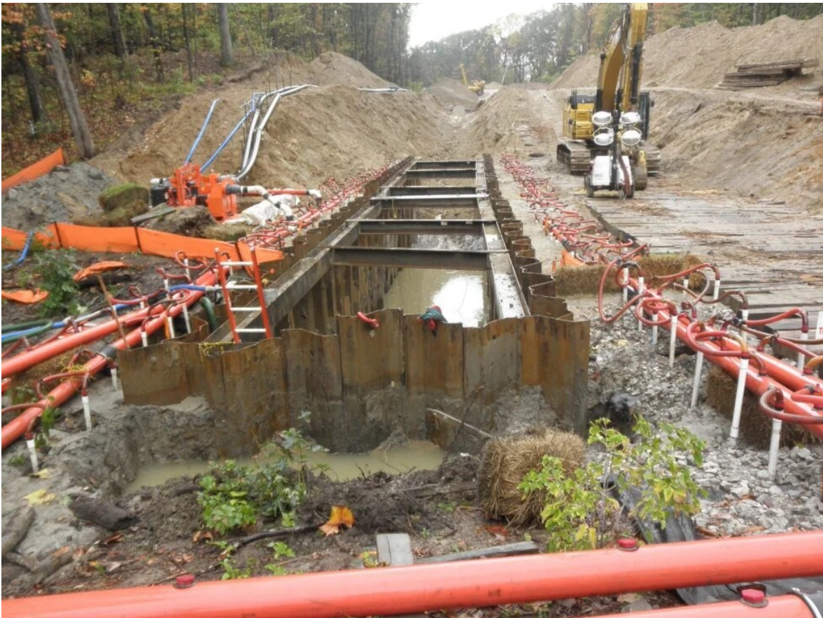
Images show: a crane and a worker installing the metal piling, and the installed piling around the pipeline trench at a dewatering site, with pumps visible.
