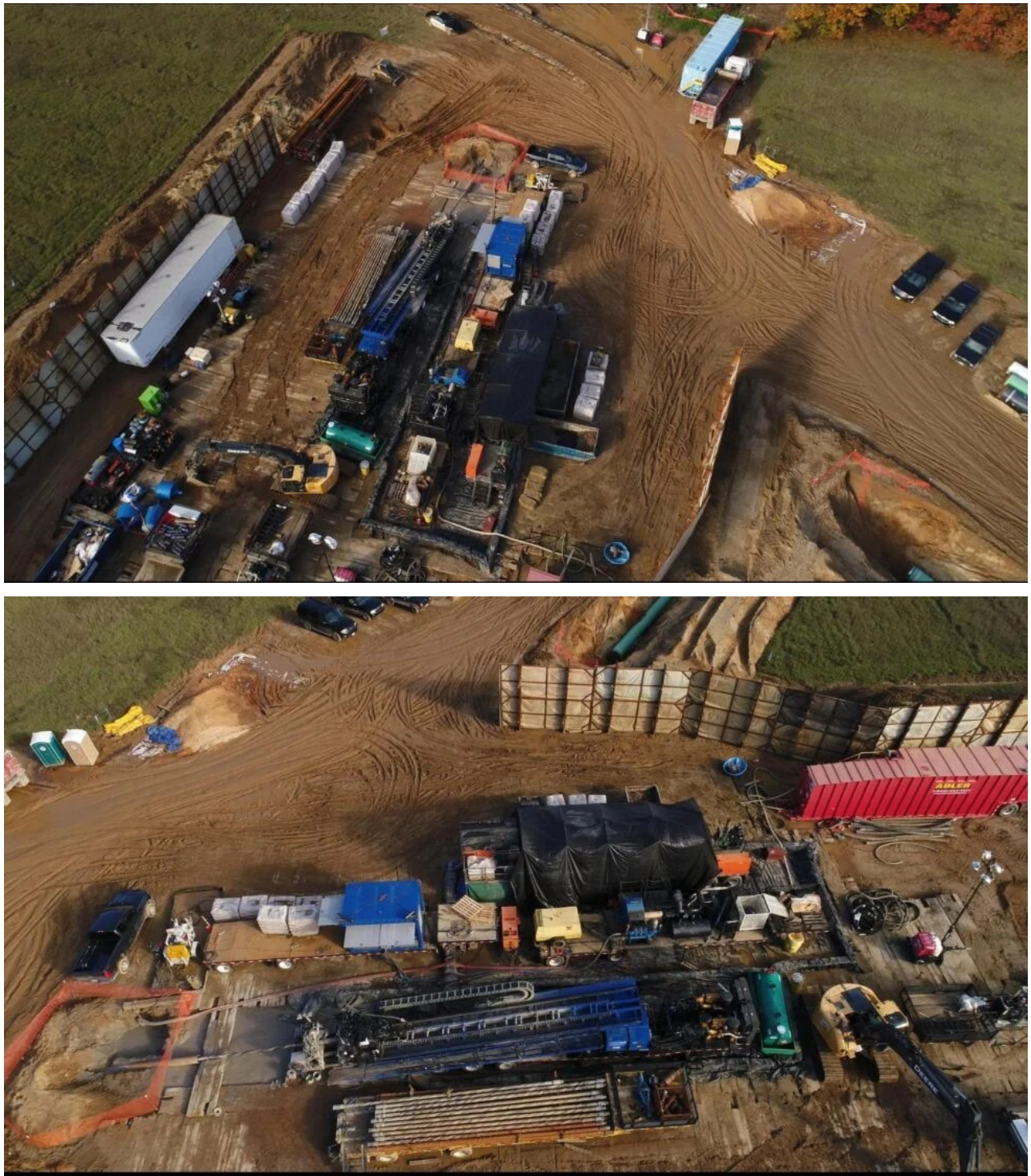
Figure 3: Images show: More drone footage of the HDD site. Note the pool holding the drilling fluid, surrounded by an orange safety fence; the blue drilling rig and the pile of drill rods next to the rig (they extend the drill bit further into the hole).
