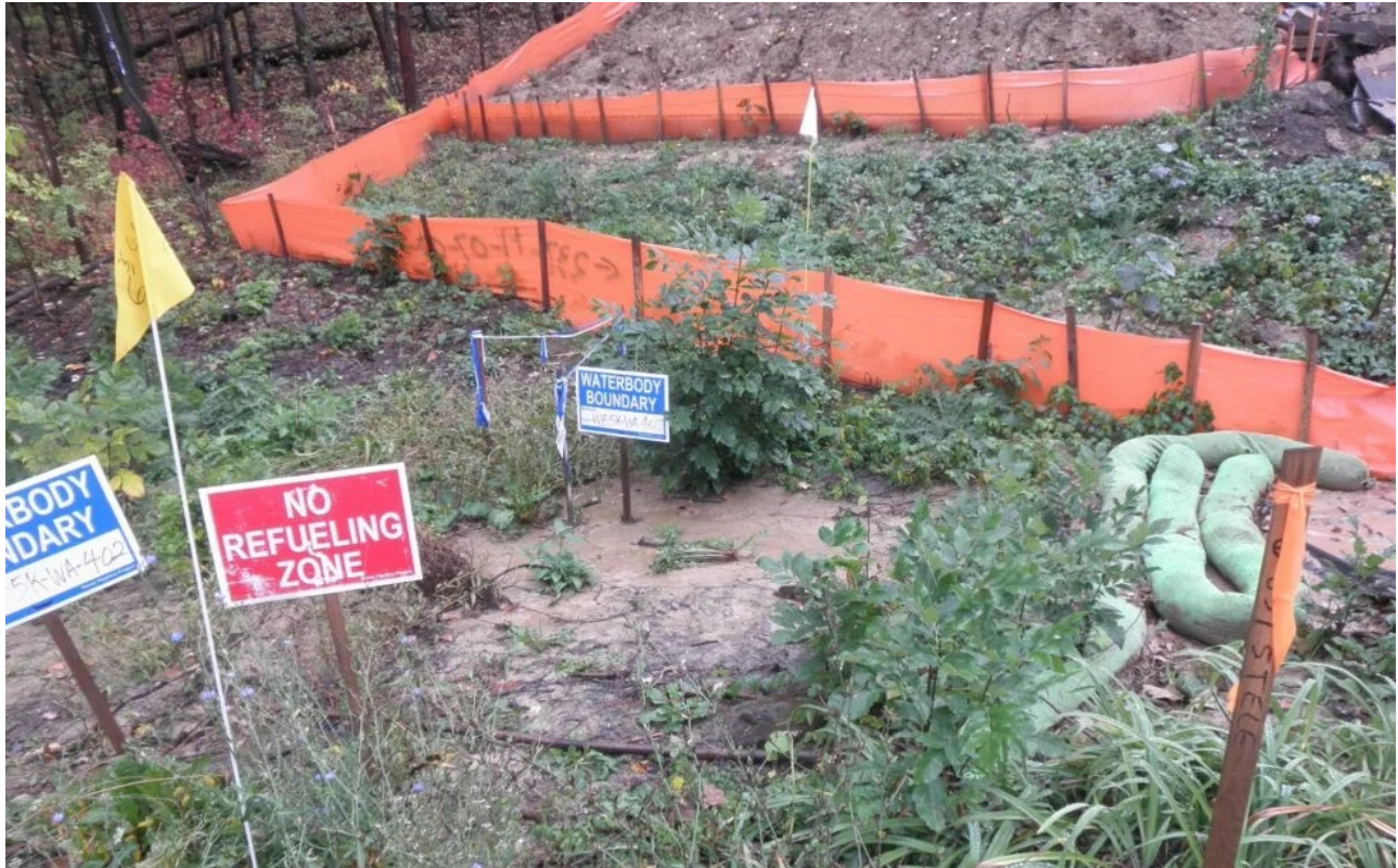
Orange sediment screens and a sand stocking installed to prevent erosion in a wetland area. Note that all the ECDs are inside the construction right of way marked by the blue and white flagging.
